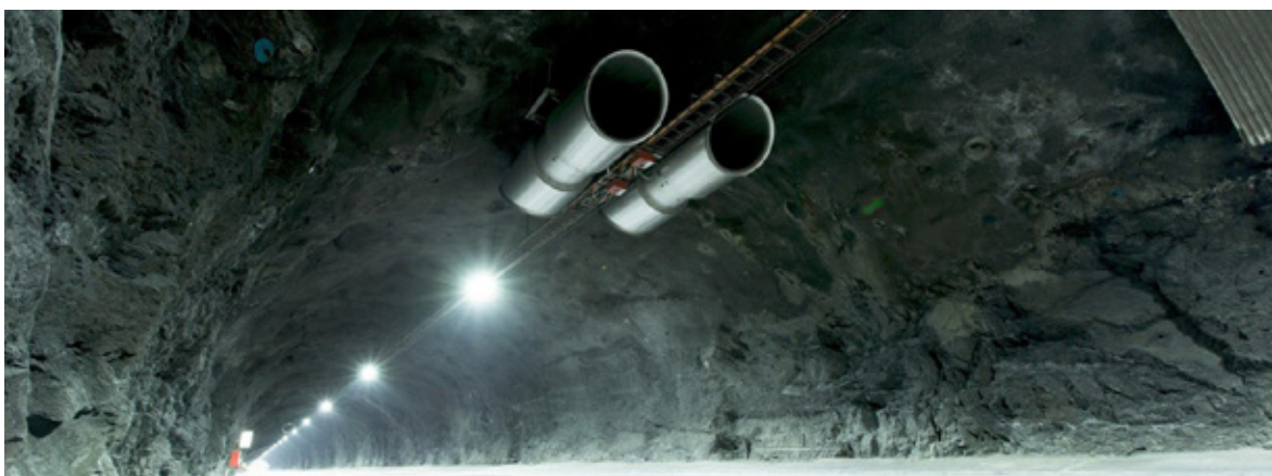
Illustration 6 - Picture of jet fans with inclined outlets.
